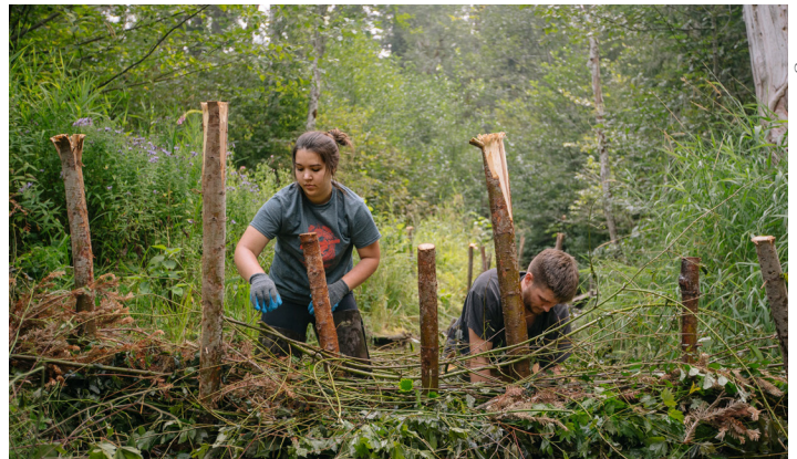
Tribes, public land managers, and others are turning to beaver mimicry and other approaches to restore riverscapes. Here, the Tulalip Tribes' Natural Resources Department installs a beaver dam analog.
