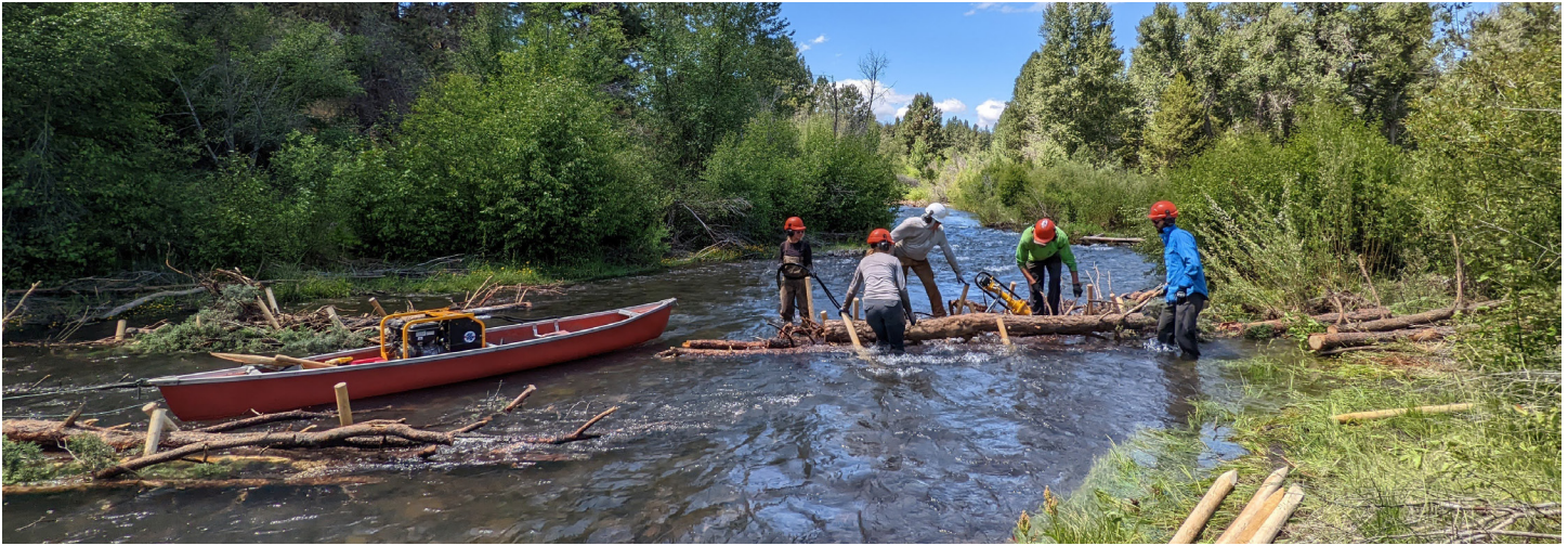
A restoration crew builds artificial logjams to slow the flow of water, capture sediment and other materials, and improve habitat.
