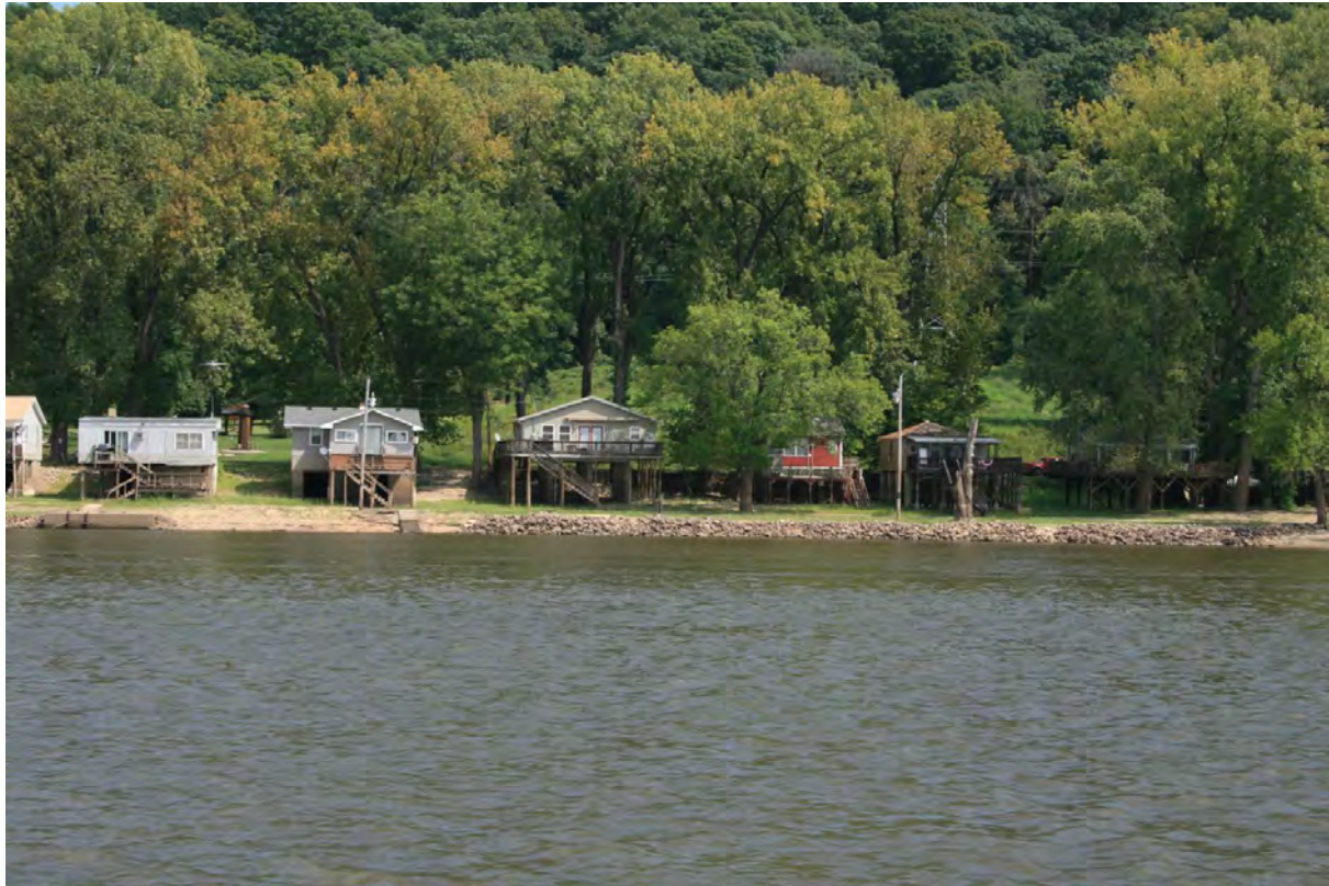
Home elevations on the Mississippi River, Illinois. Photo credit: Jenny Hoffner
