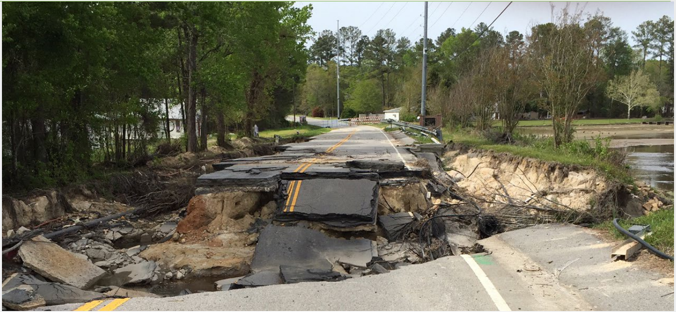
Failure of Lake Elizabeth Dam near Columbia closed Highway 21 for more than one and one-half years.
