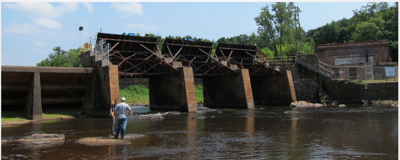
Clifton 1 Dam at Pacolet River, SC
