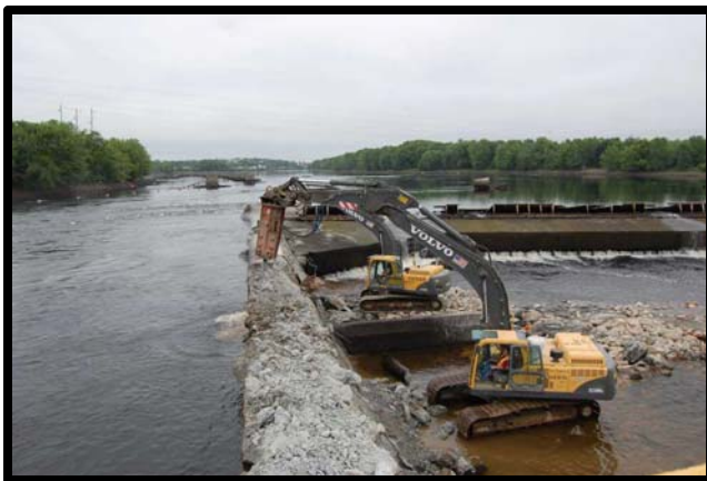
Great Works Dam removal, Penobscot River, Maine
