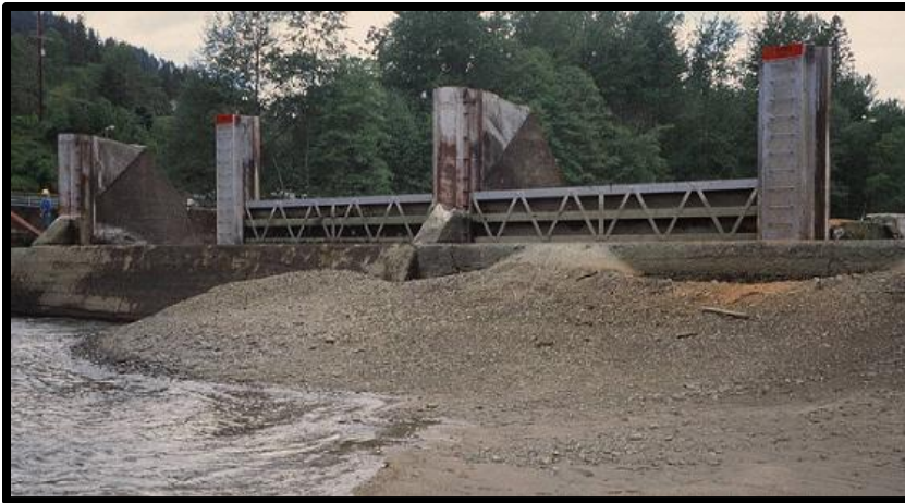
Sedimentation behind Savage Rapids Dam, Rogue River, Oregon Photo By: U.S. Bureau of Reclamation
