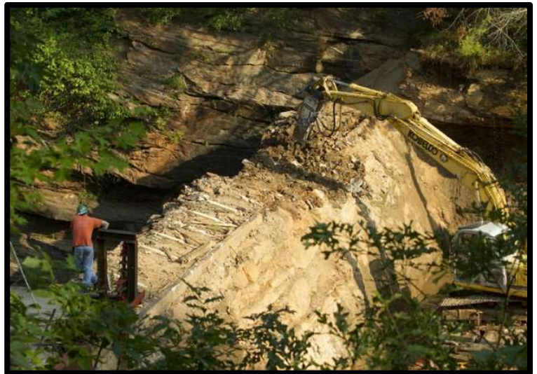
Woodside Dam II removal Twelve Mile River, South Carolina
