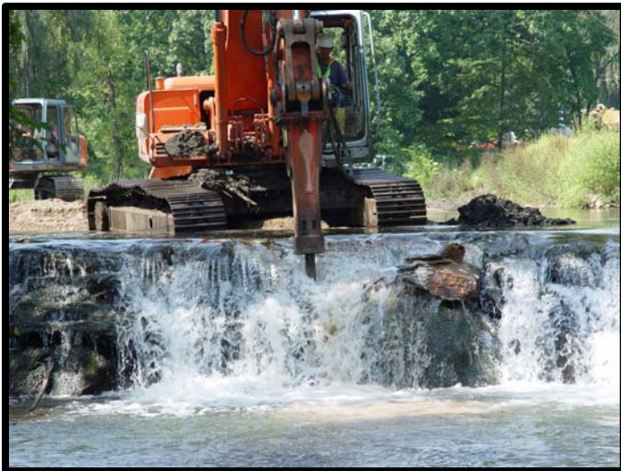
Wyomissing Creek Dam removal Schuylkill River, Berks County, Pennsylvania
