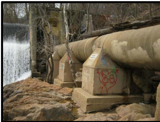
Bloede Dam Sewer Line Abutment Patapsco River, Maryland
