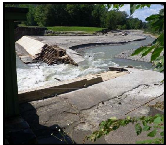
North River Dam is breached Colrain, Massachusetts
