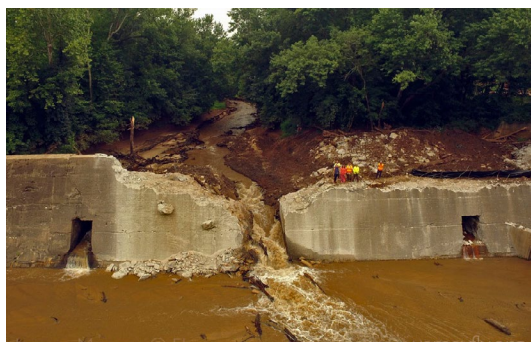
Figure 1: Shuford Dam before, during and after dam removal.
