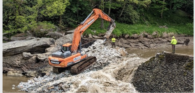
Ward's Mill Dam during construction, May 2021 Photo courtesy of American Rivers
