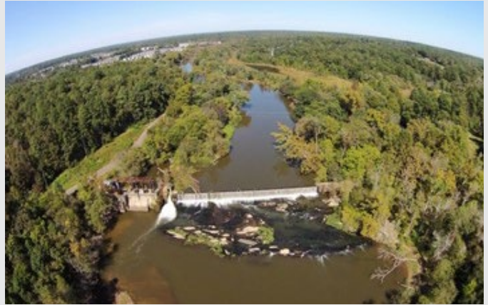
Photo of Milburnie Dam Courtesy of Restoration Systems, LLC.
